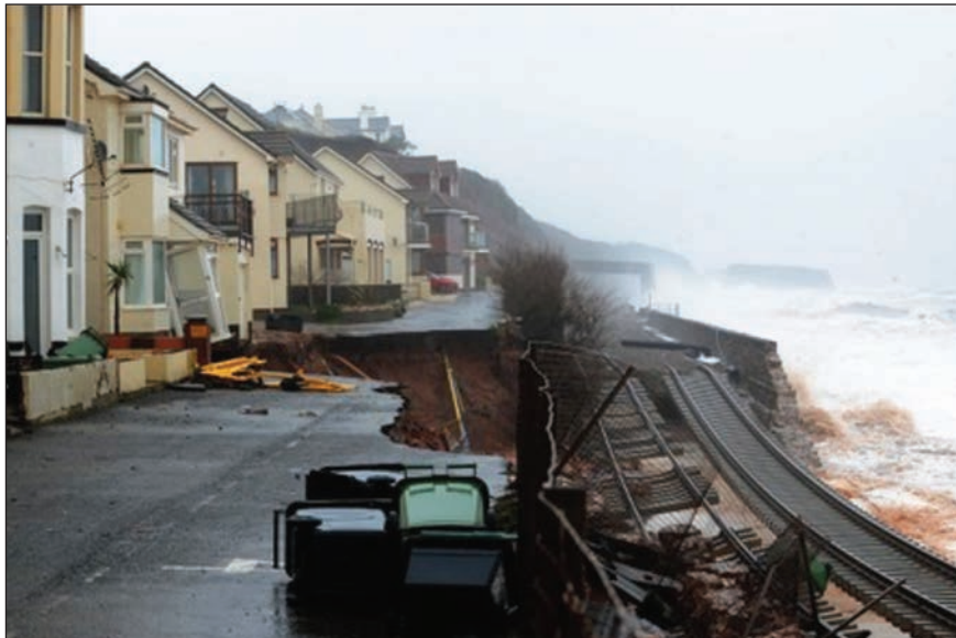
Figure 1: The impacts of high energy storm events on the coast of Devon and Cornwall during winter 2013-2014
